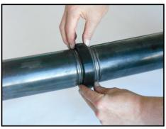
Bring the two pipe ends together edge to edge. **Ensure alignment is straight and concentric.**
