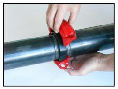
Slide the opened coupling over the pipe and over the gasket.
