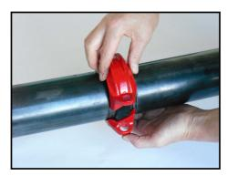
Now place the second half of the casing onto the gasket, so that the keys engage in the grooves of the pipe ends.
